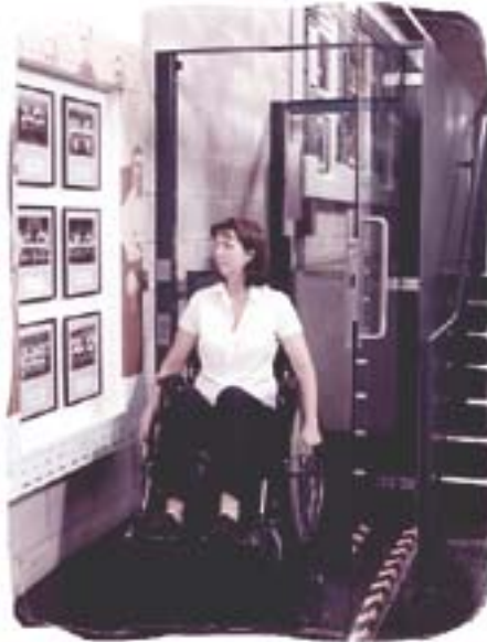
The Excel platform lift at the new National Football Museum in use.
