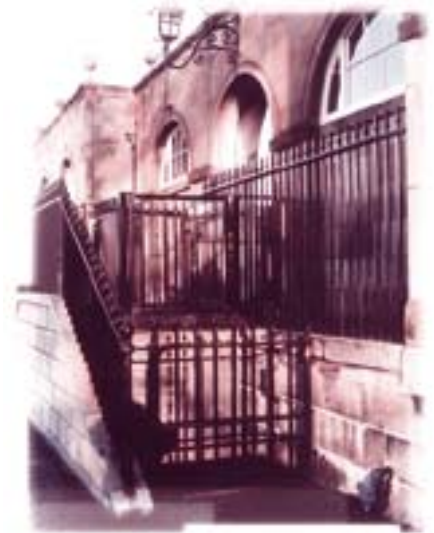
This platform lift installation shows how, with careful and sympathetic design, a platform lift can be incorporated into a building with historic interest.
