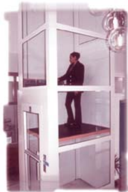
A platform lift has a platform that travels within a shaft, it has no lift car.
